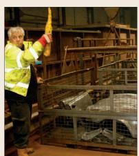
**09**Because this cleaning dip will remove all underseal and factory-applied sound deadening, the process has become very popular with race car builders. Here is a brand new Ford Focus shell that's destined to be a touring car where the extra few lbs of weight saving will make all the difference. It's a similar story if you plan to race your Mini; this is a far easier and more effective option than chiselling away at the factory sound deadening.
